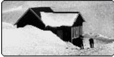
ILLAWONG LODGE incorporating Pounds Creek Hut (1925), built and run by the Club since 1956. Listed on the Register of the National Estate.
